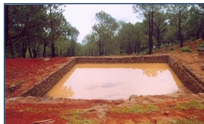
Water harvesting structure constructed
